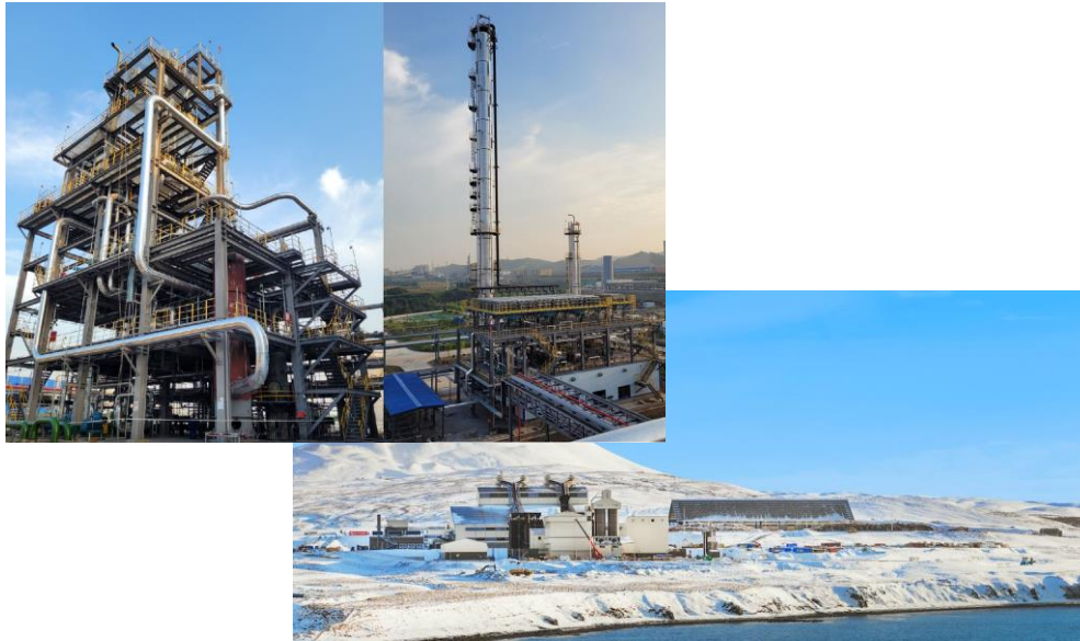
THE SHUNLI CO 2 -TO-METHANOL PLANT
